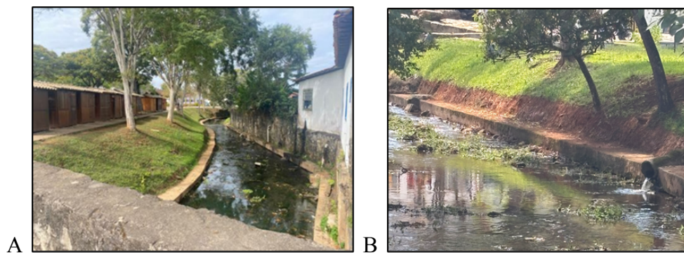
Figure 5. Santo Antônio stream in Tiradentes. Sewage collection at the stream margins was implemented in 2016 to minimize direct discharge into the stream (A). Sewage discharge into the stream in 2025, 9 years after a municipal “revitalization” project (B).
